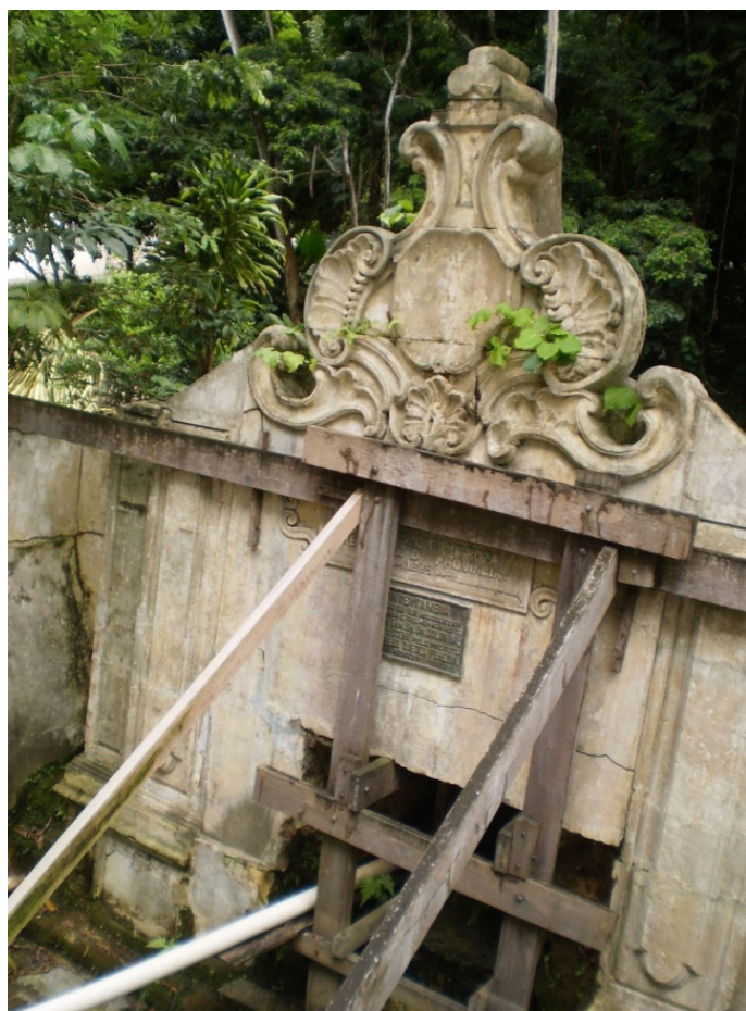
Figure 5. Degrading situation of the pediment built in the 18th century to identify the Tambiá Fountain, richly carved in limestone with baroque elements. Photo: the authors
